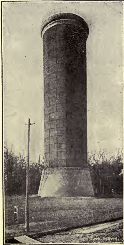
FIG. 5.—VIEW OF STAND-PIPE AT ELGIN, ILL., LOOKING NORTHWEST. ( Engineering News. )
